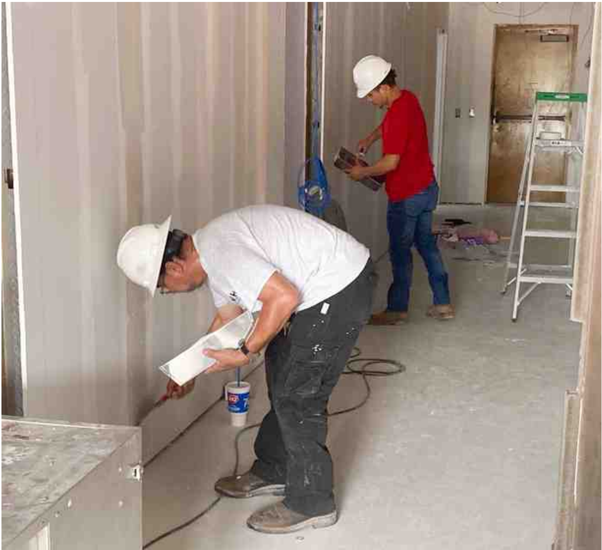
Workers installing sheetrock at the La Porte Head Start campus.
